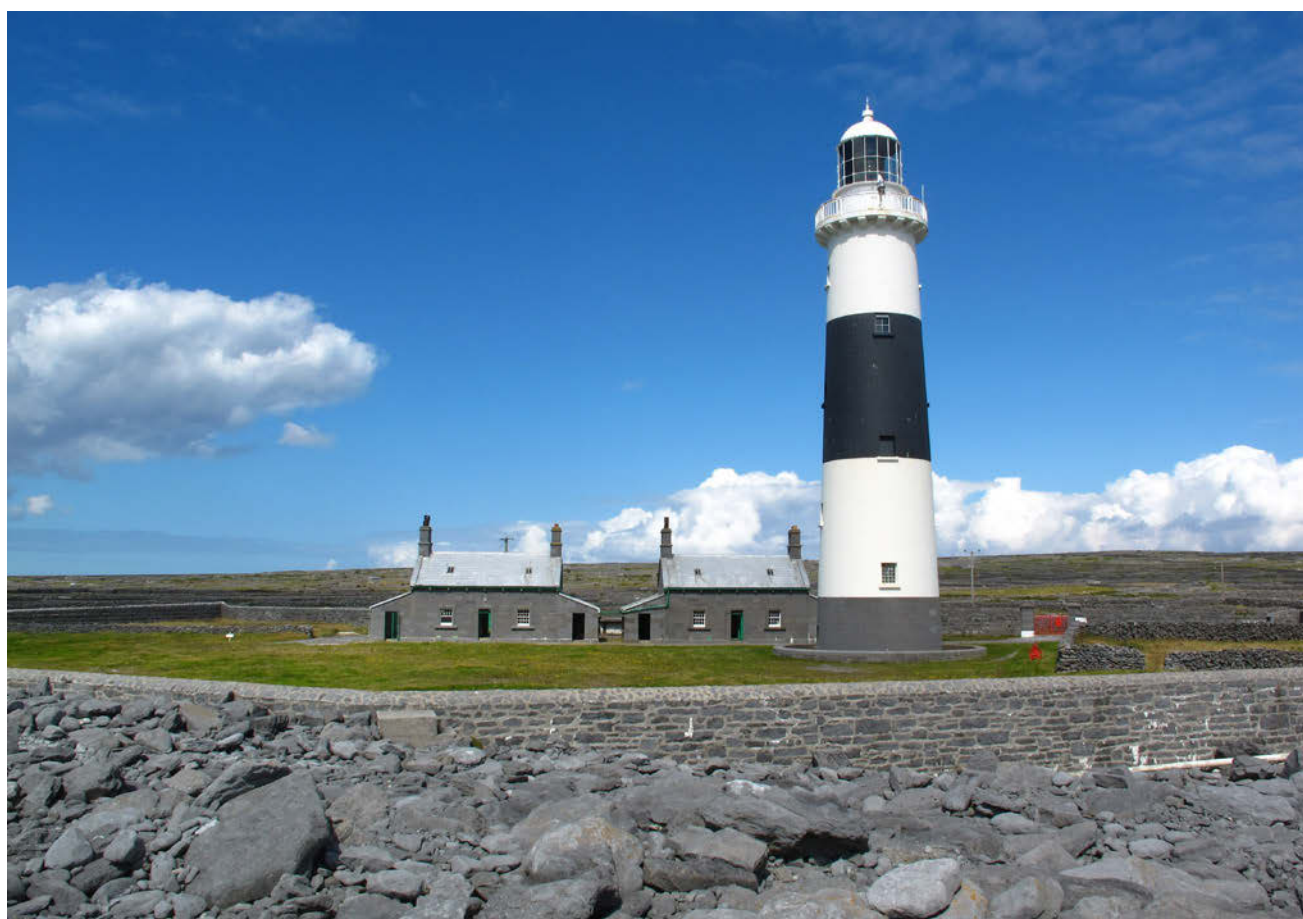
Inisheer Lighthouse, Aran Islands
