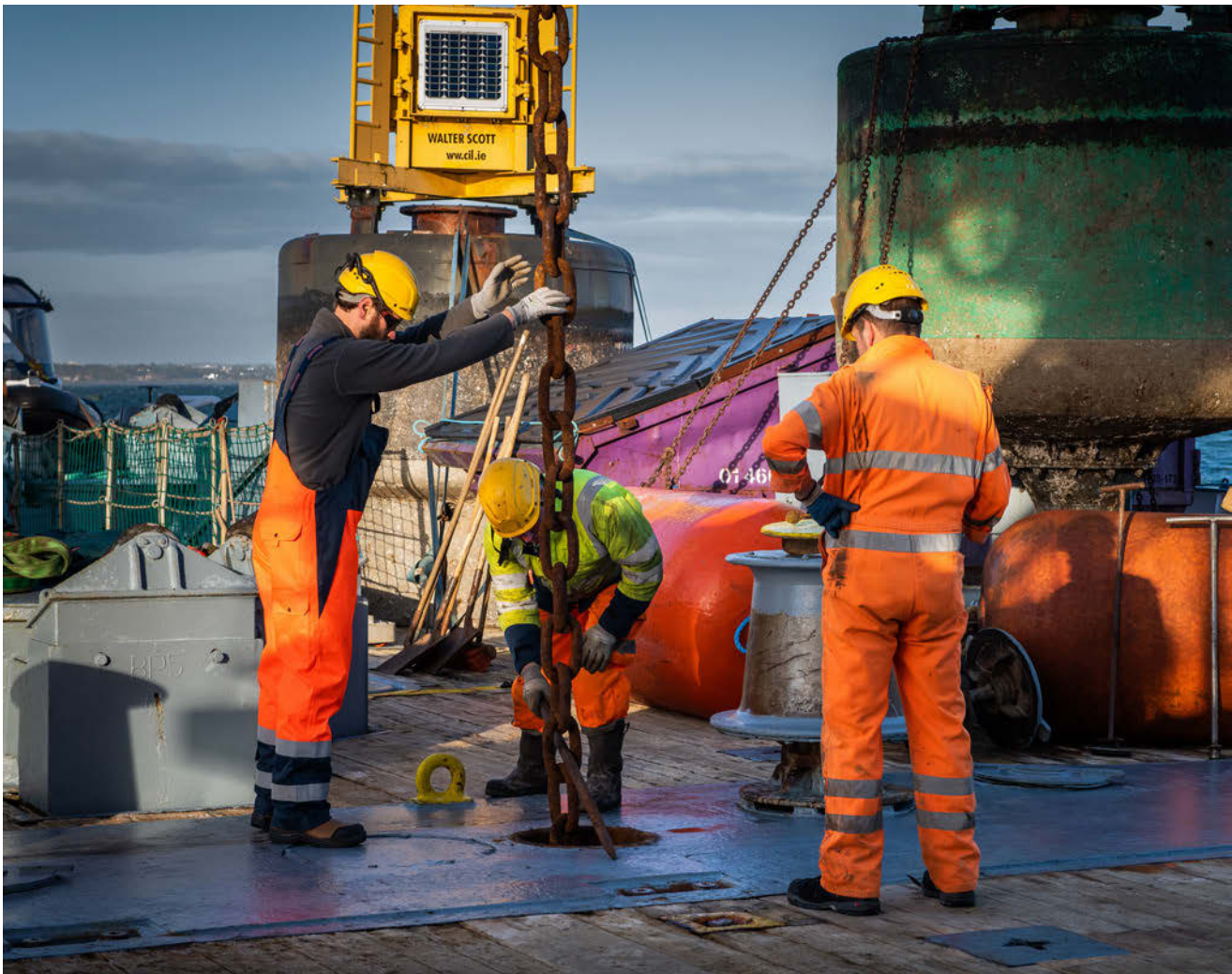
Buoy work on Deck of ILV Granuaile
